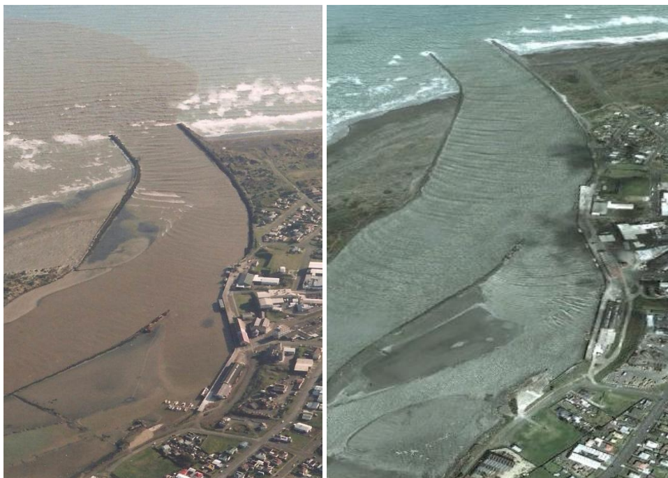
Figure 4 Comparison of the lower river at low tide in 1994 (left) with 2010 (right). The lack of a spending beach as provided by the Tanae Bank is apparent in 2010 with waves propagating into the inner harbour and up the river rather than dissipating energy by breaking (sources: Shand; left, Digitalglobe; right).
