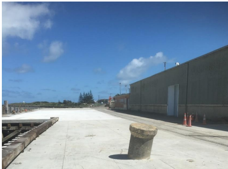
No.1 wharf deck looking west with a concrete mooring bollard in the foreground
