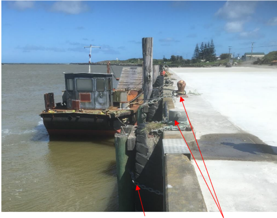
No.1 wharf face showing fendering and mooring bollards
